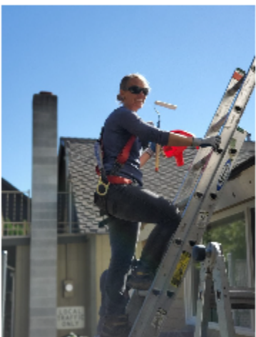
The team working on a repair project in Upper County.
